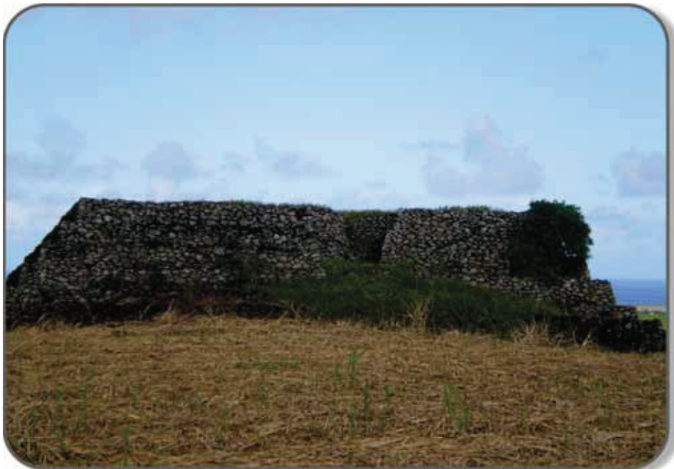
... and a damaged central portion.
