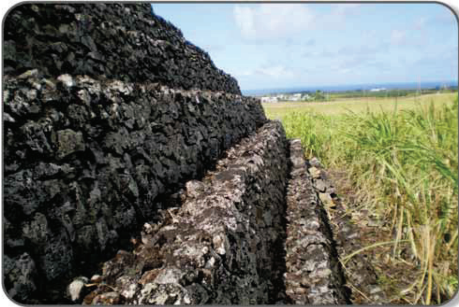
The compact construction of all seven pyramids is visible; although there is no bonding material, the structures have remained preserved for a long period of time due, I believe, to the mastery of their ancient builders.
