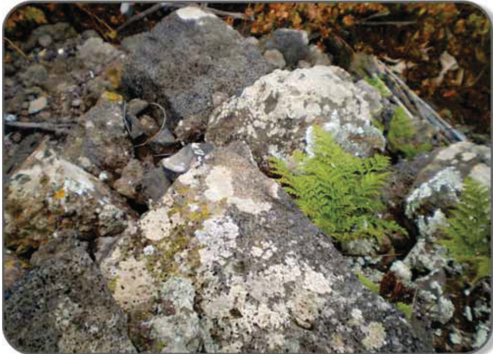
Pyramid corners are built from the shaped corner stones.
