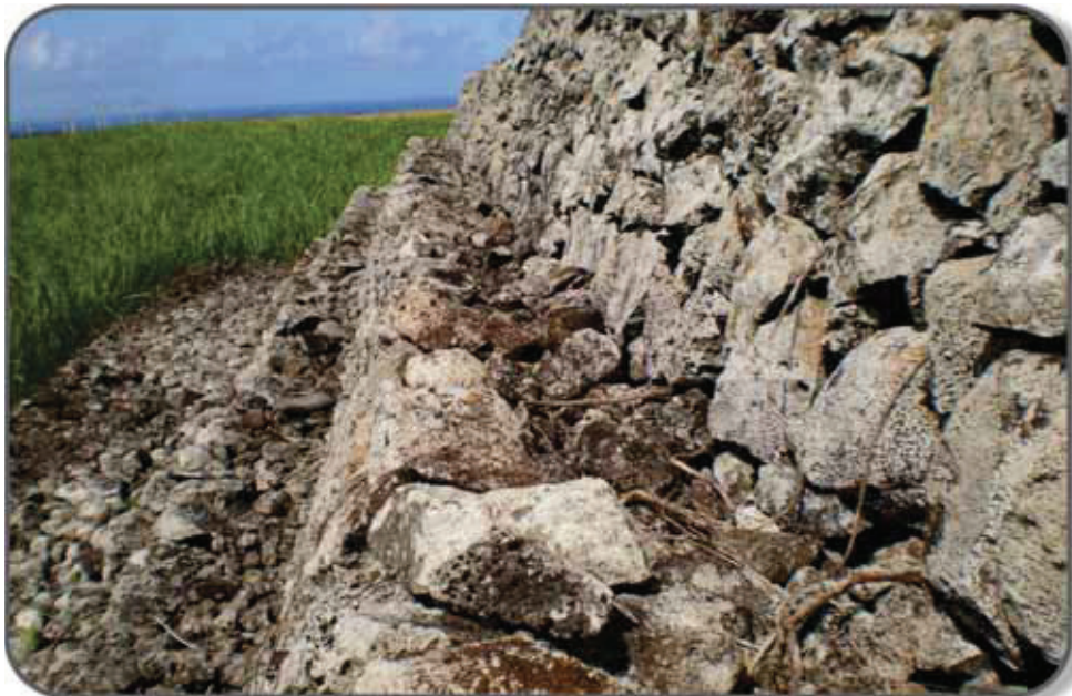
The same building system is implemented at all steps at Mauritius: Larger volcanic stone lines the edges, and smaller stones fill in the internal sections
