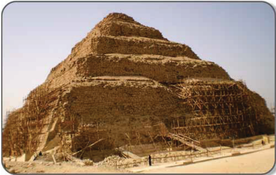
Scaffolds on all four sides of Step Pyramid
