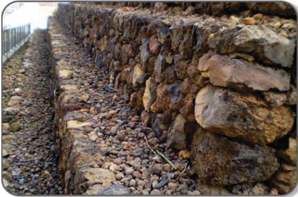
Pyramid No. 5 combines same size volcanic rocks at the pyramid edges, volcanic gravel inside and shaped corner volcanic stones. A planned approach is obvious.
