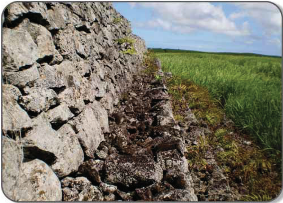
The internal slope contributes to the stability of the building. The east side of each pyramid is oriented toward the Indian Ocean.
