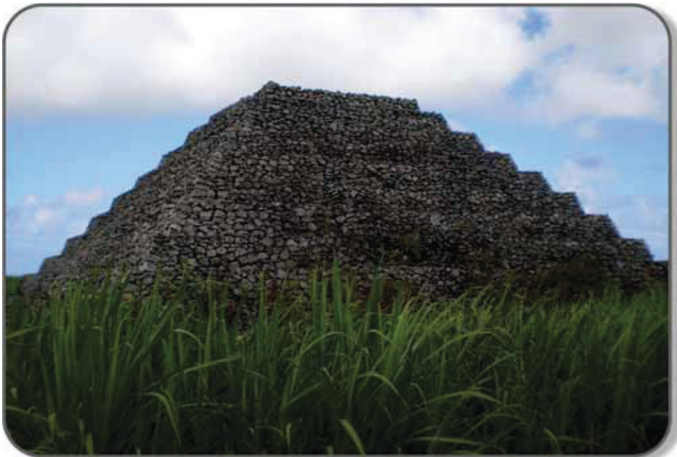
Pyramid No. 5, so-called the "white pyramid" because it's made from lighter-colored volcanic stone, consists of 11 steps and has a square base of 24.95 x 24.95 meters
