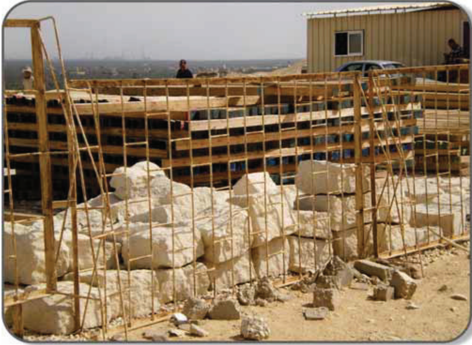
Stone blocks ready for installation in the Step Pyramid
