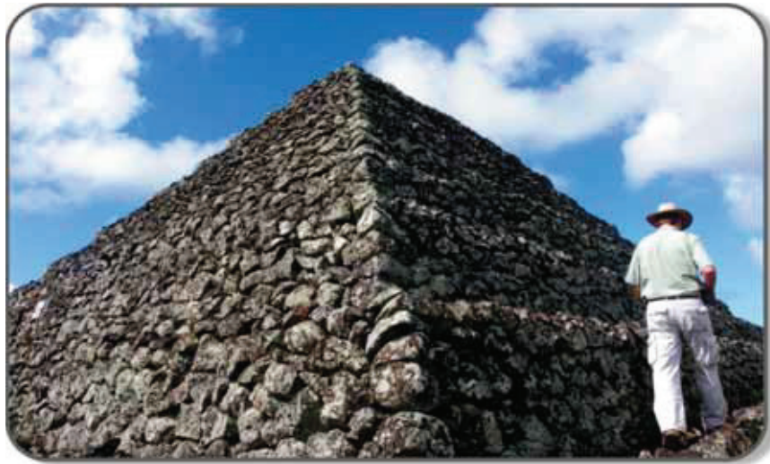
Pyramid No. 1 in Mauritius has properties identical to the pyramids in Guimar, at Tenerife; shaped volcanic stone was used as a construction material; corner stones were shaped on both sides; pyramid triangular face is oriented towards the east
