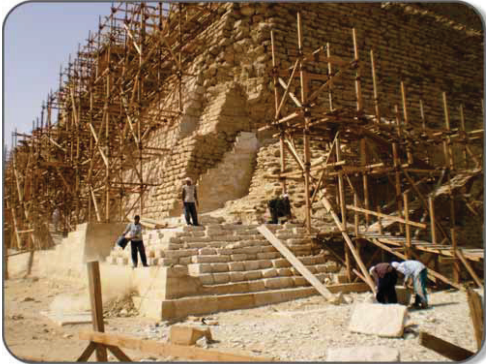
Reconstruction of the Step Pyramid at Saqqara partially distorts the original geometry of the pyramid
