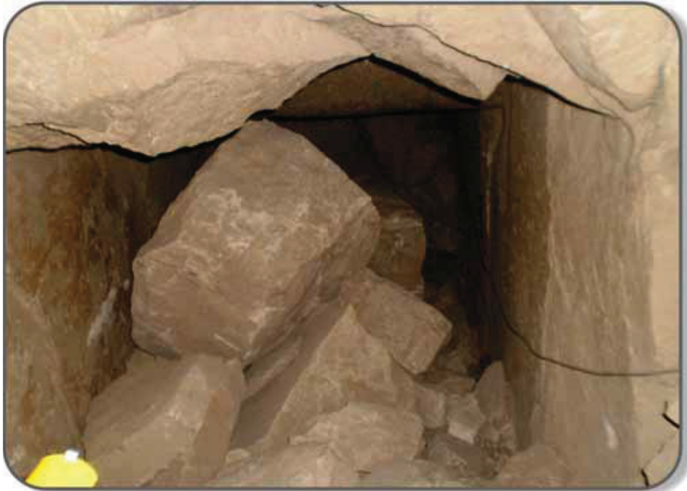
Collapsed arches in the interior of the Pyramid Sahura
