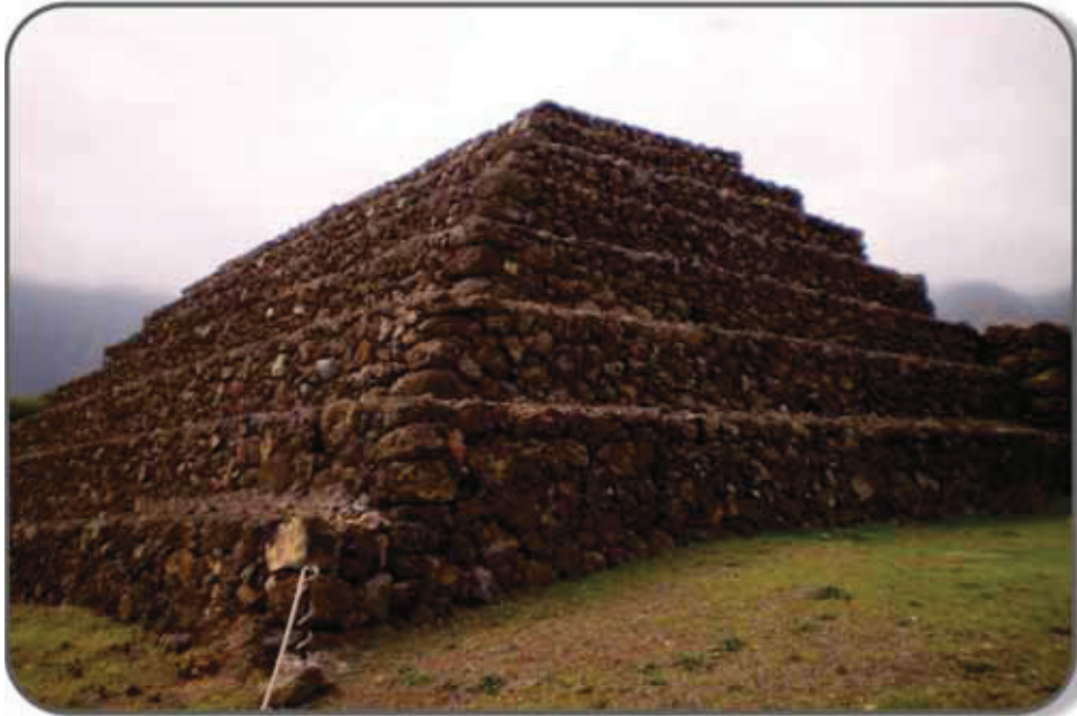
Pyramid No. 1 in Guimar, at Tenerife island, has identical characteristics like the pyramids in Mauritius; volcanic stone is used as a construction material, corner stones are shaped at 90 degree edges, orientation is to the east.
