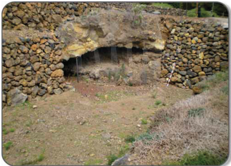
The tunnel passage in the volcanic rock beneath the western side
