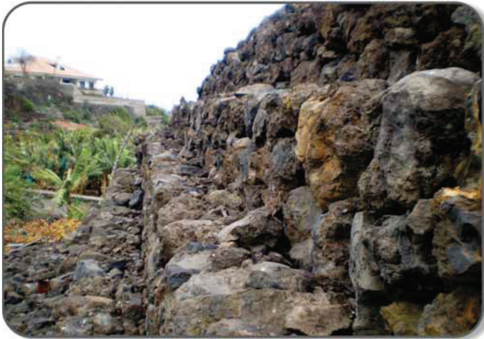
Same-size shaped volcanic stones have been used for the pyramid steps.
