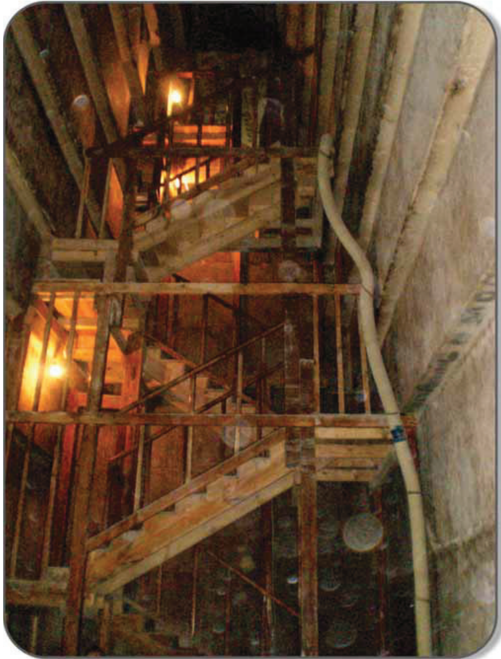
Improvised stairs lead to the third gallery inside the Red Pyramid
